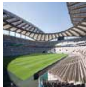
Location_Korea Project_Soccer Stadium
