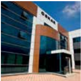
Location_Turkey Project_Office building
