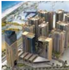
Location_U.A.E Project_Residential Building
