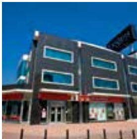
Location_Turkey Project_Office Building
