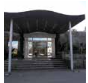
Location_Slovenia Project_Utility Company
